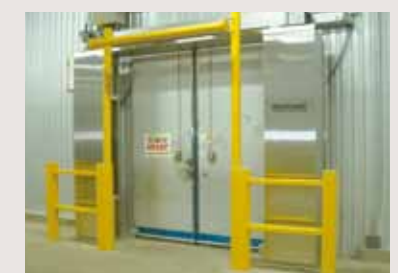
Cold storage Inside -25°C / Outside -5°C Size: 2,600mm (h) x 2,200mm (w) Door opening by Pull switch
